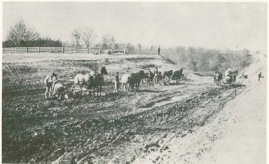
The western end of the big cut and fill. In that the steam shovels were tied up on the bigger cut to the east, the western cut was made primarily with hand labor and dump carts. This photo was taken from the approximate location of the Soo Line crossing at Meadow Lane.
