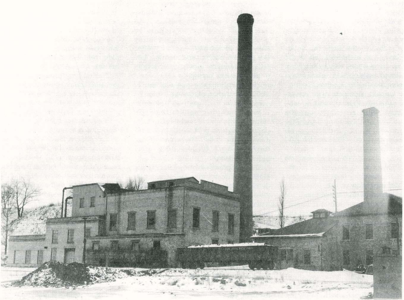
Manitowoc Public Utilities pumping station generator room and boiler house (at left) constructed in 1916 during Henry Stolze's second term as mayor. Note that Lincoln High School is not yet constructed on Roeff's Hill in the background. The present Manitowoc Public Utility is located in the same location where the Stolze Administration constructed its new facility. The city today takes great pride in the efficiency and quality of its service. Although municipal ownership of city water service became the norm and still is today, Stolze went farther and acquired the city's electric franchise also. Thus today's Manitowoc residents enjoy the fruits of Henry Stolze's reforms as the city's electric rates are among the lowest in the state.
